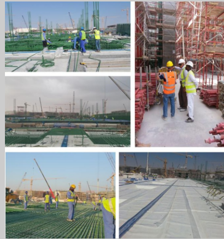
(CCC) KAHRAMA WATER MEGA RESERVOIR PROJECT - PACKAGE A (PRPS-1) UMM BIRKA
