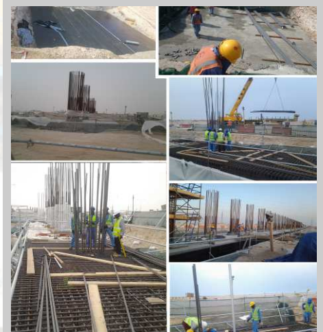
WAKRA BY PASS PROJECT L&T SITE @ WAKRA
