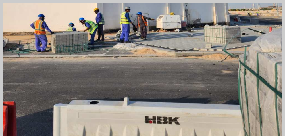
HBK - ROAD & INFRASTRUCTURE AT UMM-SALAL 2 PHASE
