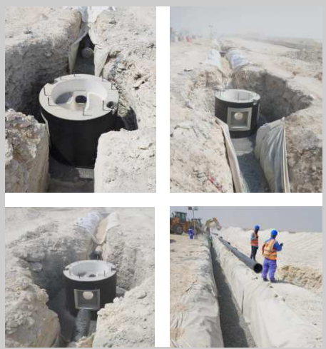
PIPE LINE PROJECT LUSAIL
