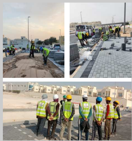
HBK - ROAD & INFRASTRUCTURE AT UMM-SALAL 2 PHASE
